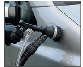
▶ Sandblasting agent is extracted and returned immediately after hitting the surface
